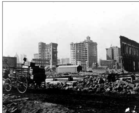
Figure 7. Massive earthquake and fire damage in San Francisco, San Francisco Earthquake (magnitude 7.8), April 18, 1906. The fire resulting from the earthquake was a major contributor to the losses. Photo courtesy of USGS ( www.usgs.gov ).
