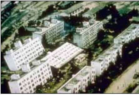
Figure 1. Damage due to soil liquefaction in apartment buildings in Niigata, Japan, Niigata Earthquake (magnitude 7.5), June 16, 1964. Liquefaction is a phenomenon that happens when the strength of saturated soil is reduced by the earthquake's sudden movements and as a result the soil behaves like a heavy liquid. Photo courtesy of NGDC ( www.ngdc.noaa.gov ).
